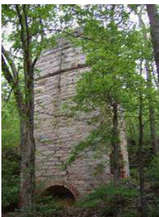
Rockwoods Lime Kiln
